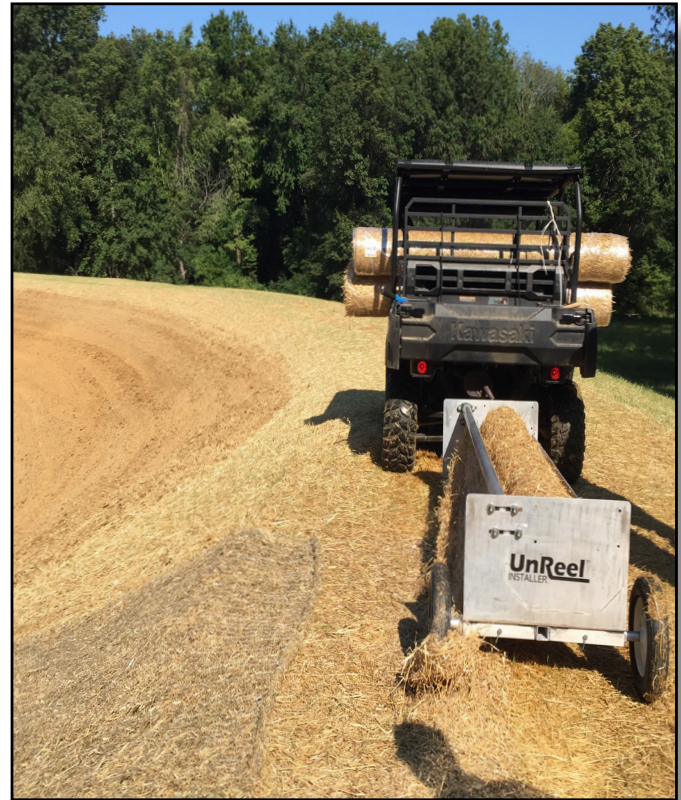
When placed at top of slope, the UnReel Installer easily facilitates the unreeling of RECPs down steep and or long slope stretches. No top of site slope access? Place at bottom of slope for upslope unreeling.
